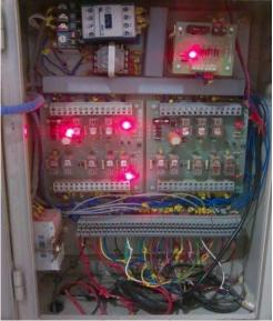
**Fig(3):** controlling part of conventional elevator
