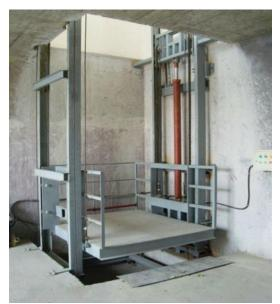
Fig(1): Hydraulic Elevator
